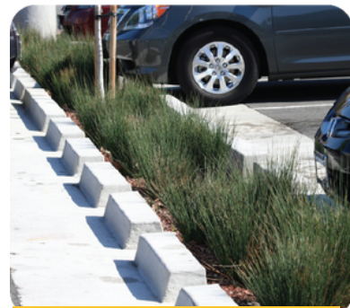
Bioswale detail in parking area
