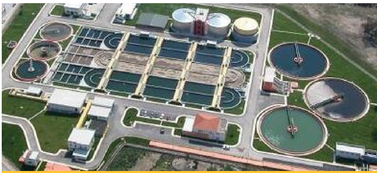
Centralised wastewater treatment plant
